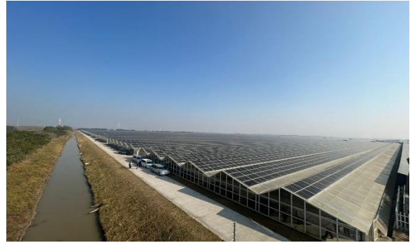
The rooftop solar energy system fully generates the energy needed for the farm and center's operations
