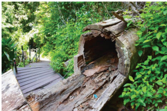
Fig. 2a. A large tree was fallen and damaged the walking pathway.
